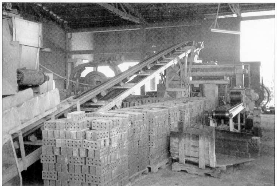
Figure 4 Medium scale factory using mechanized methods of mixing and moulding bricks
