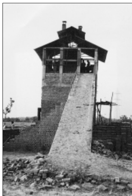
Fig. 2: The Datia kiln after opening up the operation room on top.
