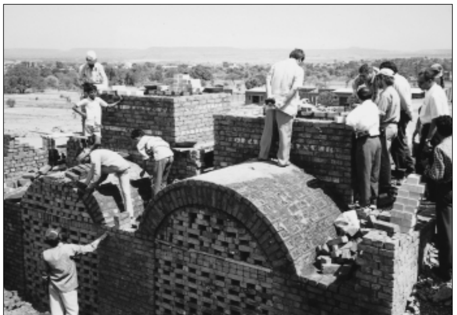
Fig. 5: VSBK-4 in Pune under construction.
